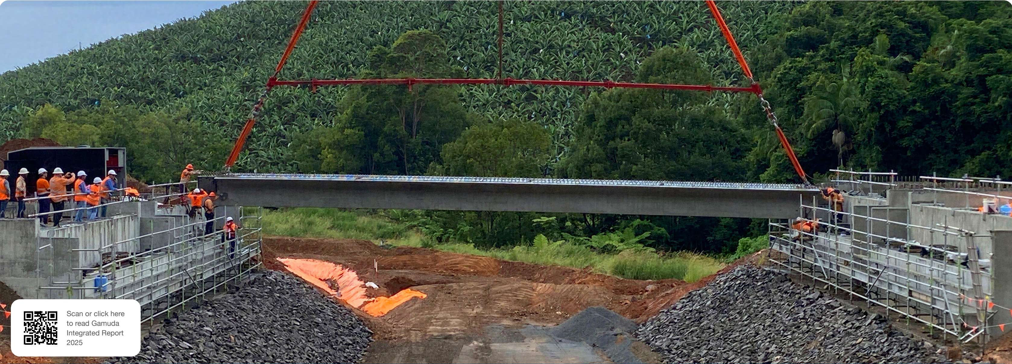
Super-T girders successfully installed over Mackays Road just before Cyclone Alfred in Coffs Harbour, New South Wales, Australia — thanks to precise planning, teamwork and a strong focus on safety.
