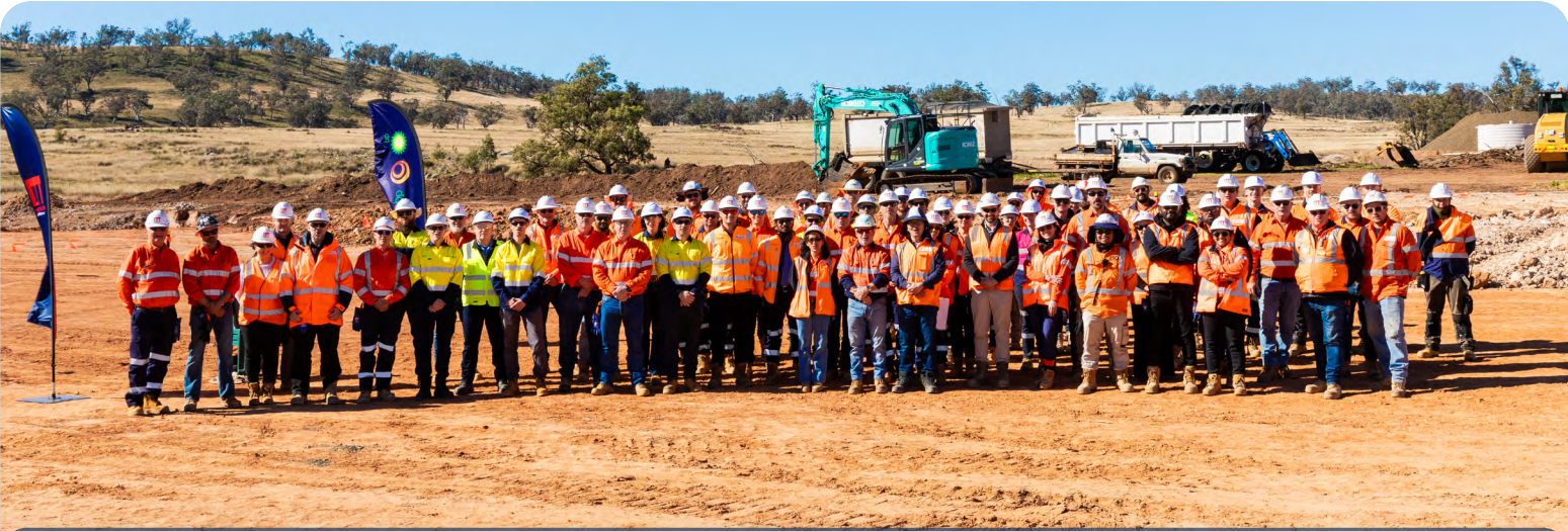
Goulburn River Solar Farm construction site, New South Wales, Australia.
