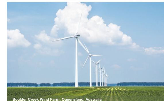
Boulder Creek Wind Farm, Queensland, Australia
