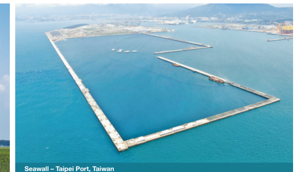
Seawall - Taipei Port, Taiwan
