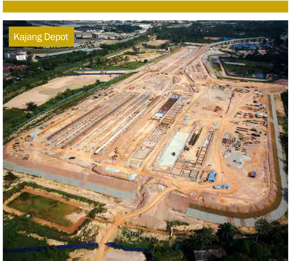
Building foundation, concreting and structural formwork in progress for the 60-acre Kajang Depot.
