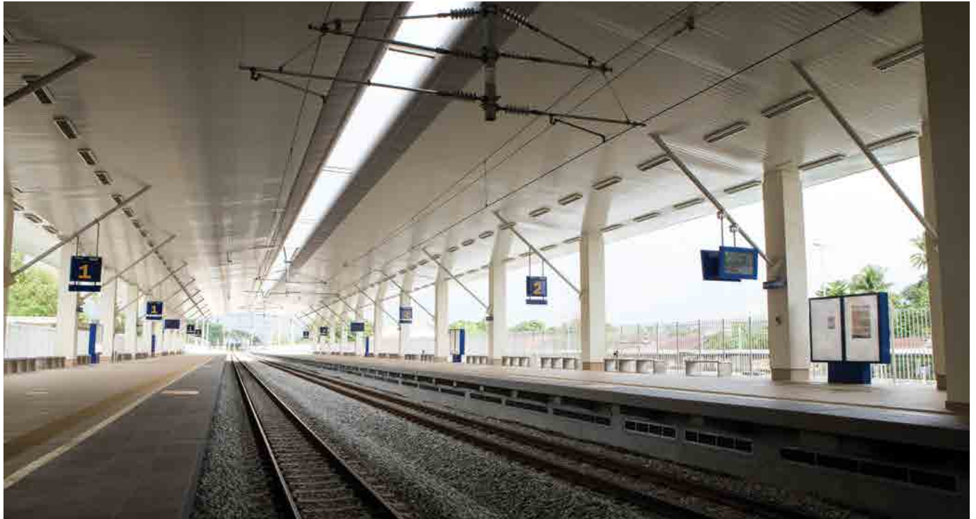
An inner view of the royal station in Kuala Kangsar, Perak. It is one of the major stations that consist of 300m length of platform as compared with other stations, 150m.
