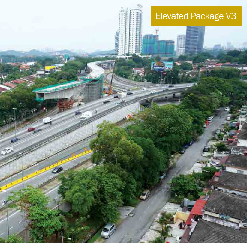
Challenging construction of MRT biggest pier heads located at the intersection of Jalan Damansara and LDP Highway (beside Taman Tun Dr Ismail, TTDI).
