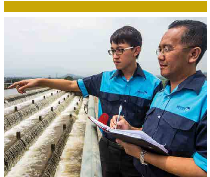
The water aeration process increases the oxygen level to eliminate bad odour from raw water.
