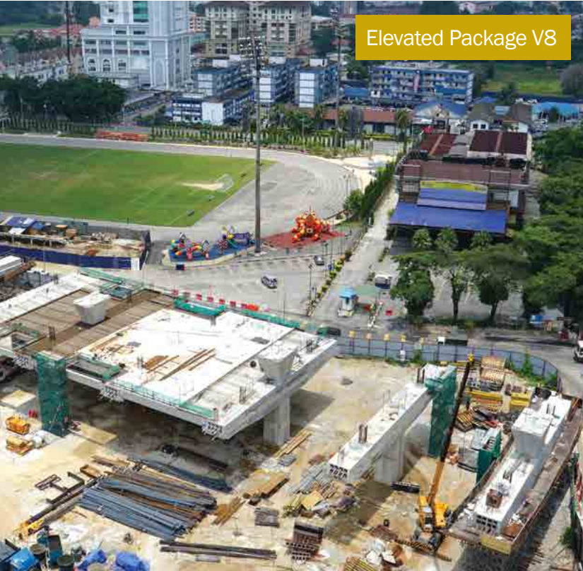
Ongoing concourse T-beam and pier head construction at the future Bandar Kajang MRT Station, as the alignment runs along the Kajang Stadium.
