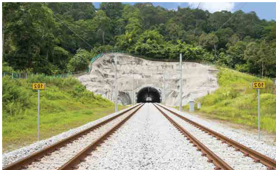
The completed 343m Larut Tunnel in Perak.
