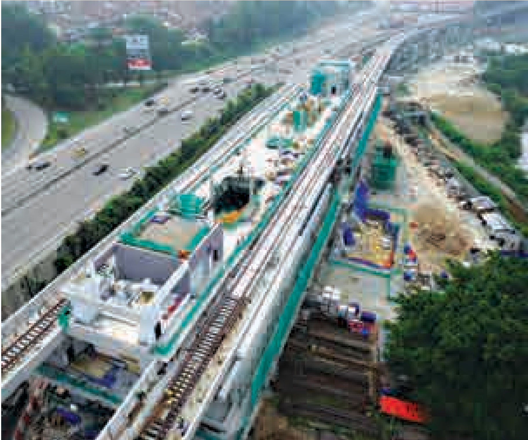
Station works in progress at the Taman Suntex Station.
