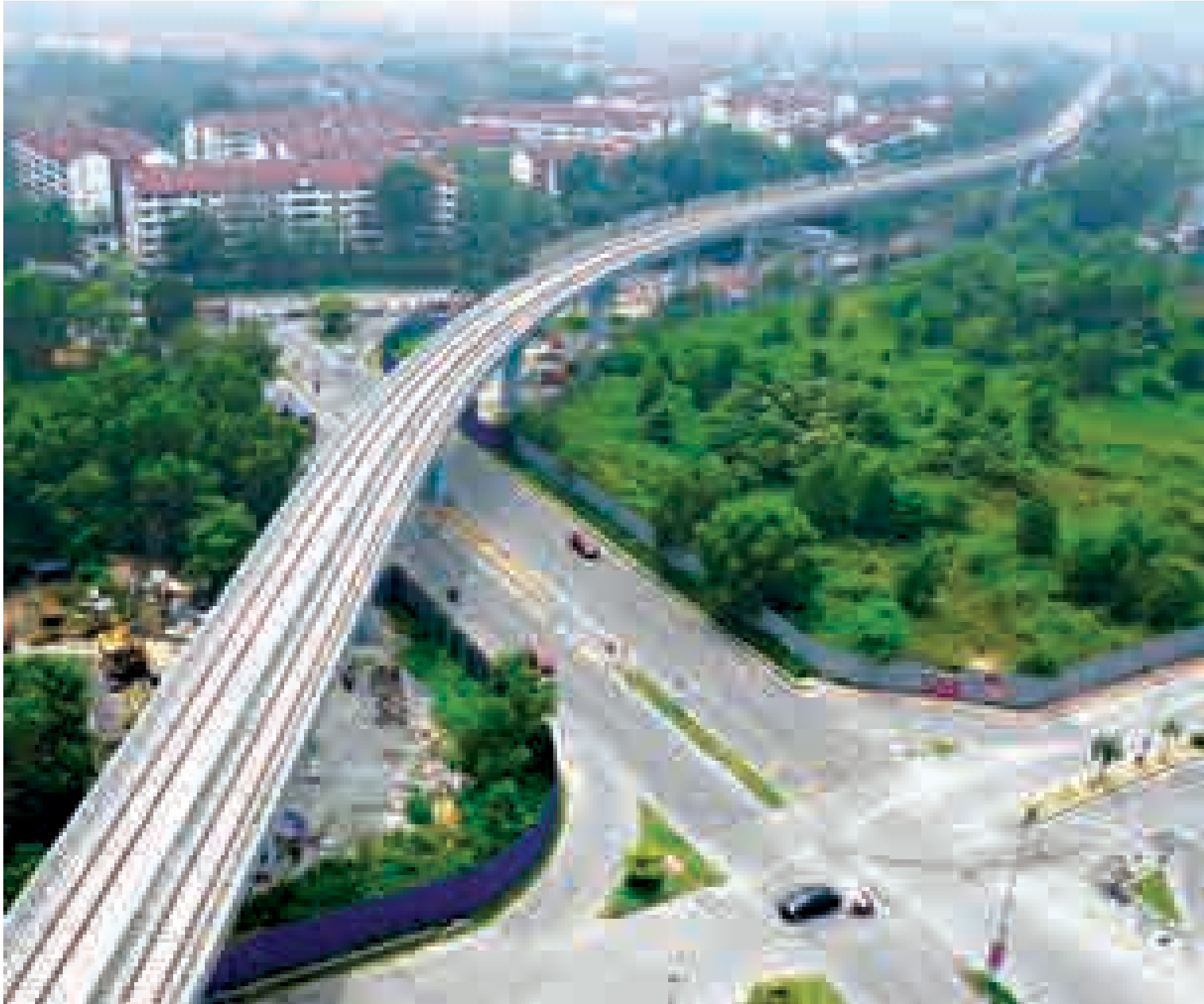
Completed track works as the alignment traverses past Kota Damansara.
