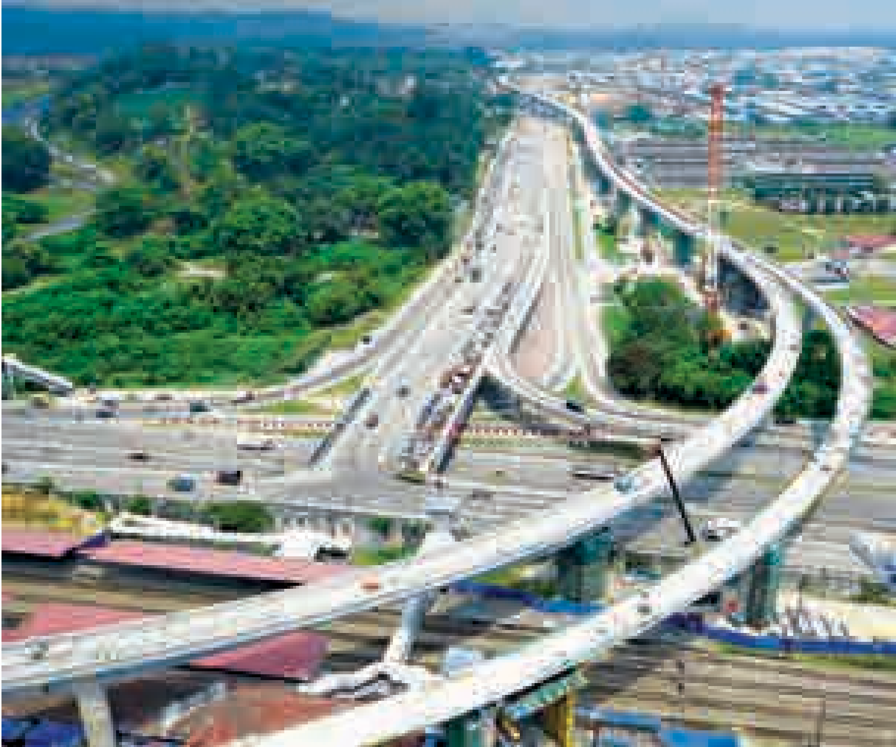
The completed 129m span across the busy Jalan Kuala Selangor, leading towards the Kampung Selamat Station.
