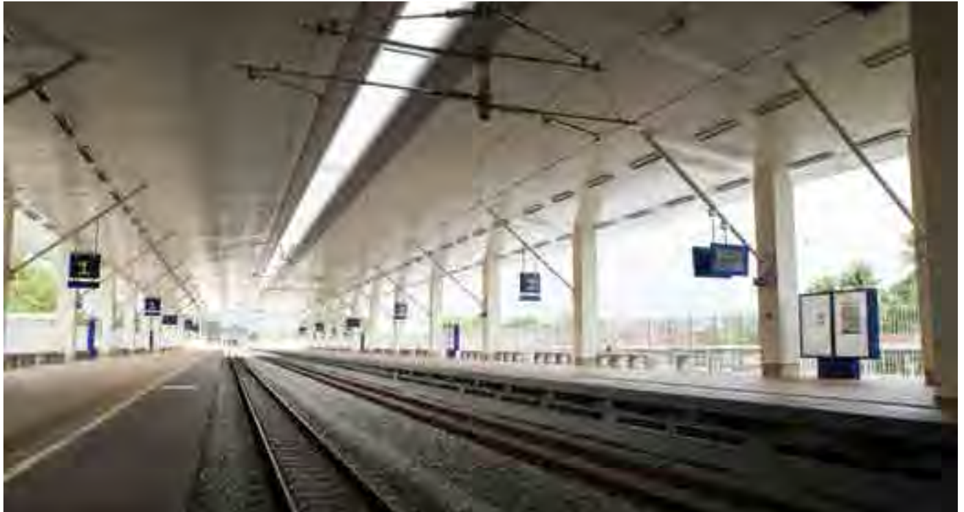
An inner view of the royal station in Kuala Kangsar, Perak. It is one of the major stations that consist of 300m length of platform as compared with other stations, 150m.
