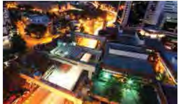
Future Semantan MRT Station for Klang Valley Mass Rapid Transit (Sungai Buloh - Kajang Line).
