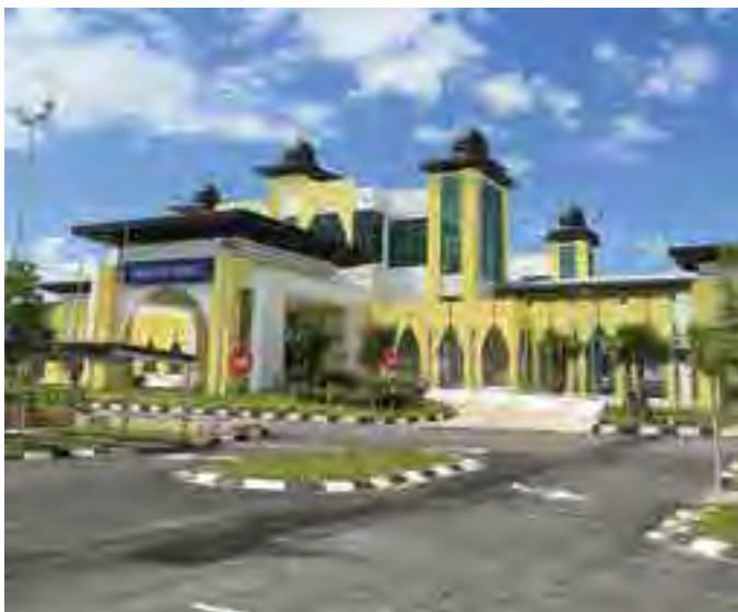
One of the completed royal stations in Anak Bukit, Kedah.
