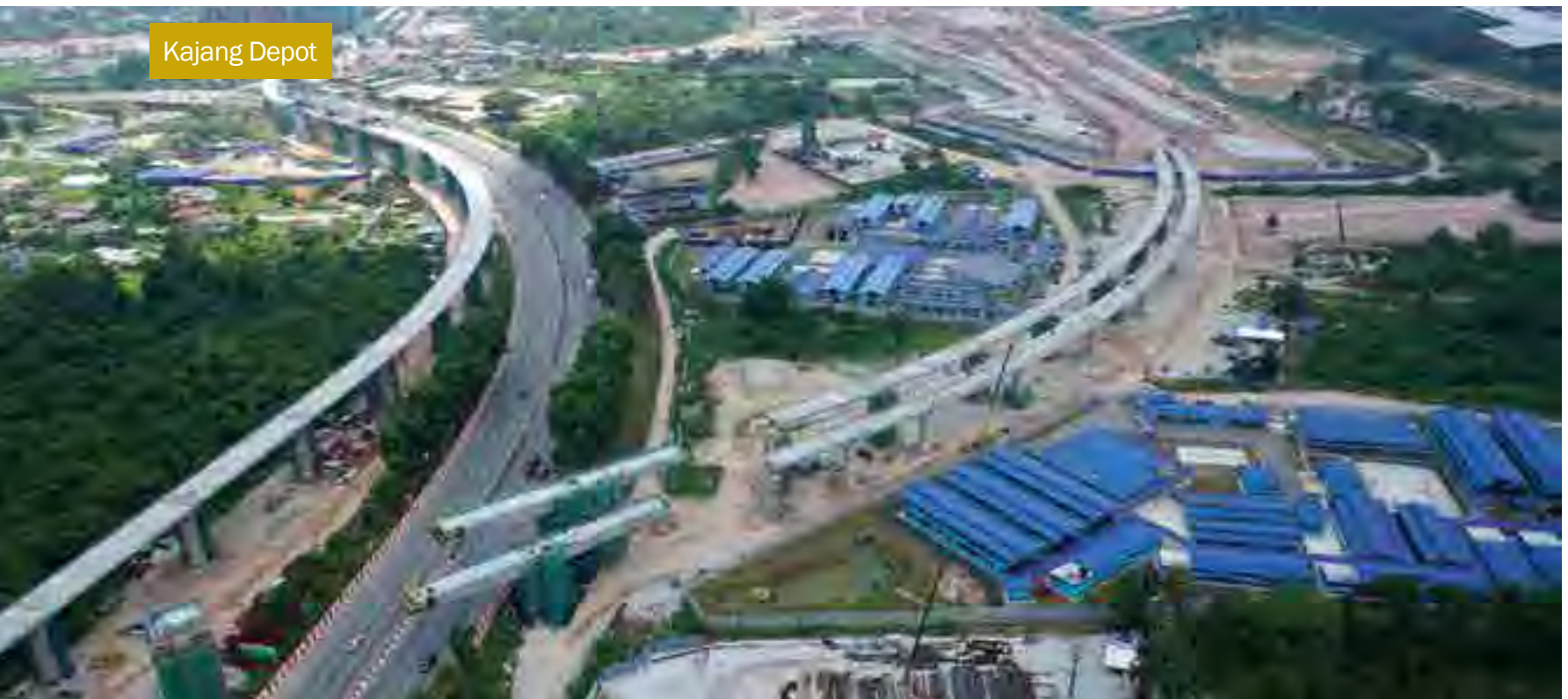
MRT guideway construction in progress for special span crossing the Cheras-Kajang (Grand Saga) Highway, leading towards the Kajang Depot and CLQ for V7 and V8.
