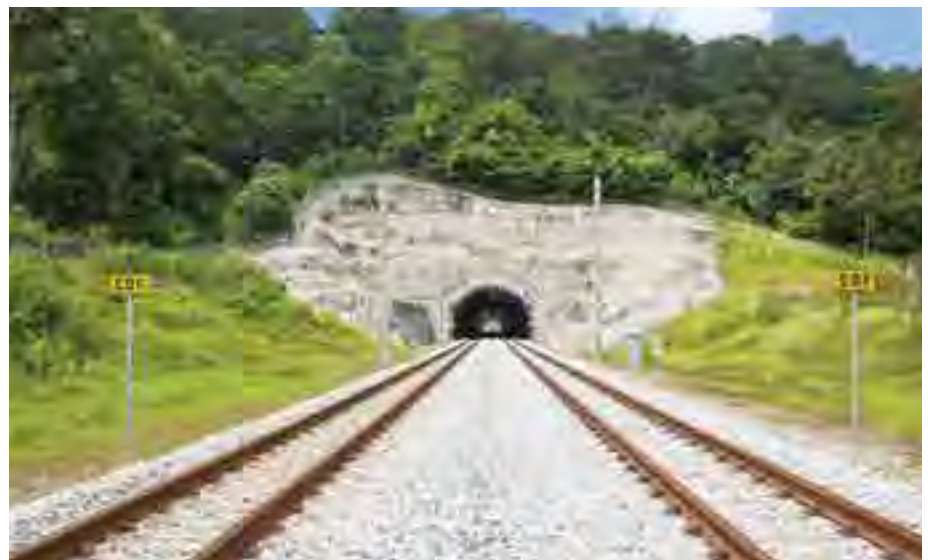
The completed 343m Larut Tunnel in Perak.
