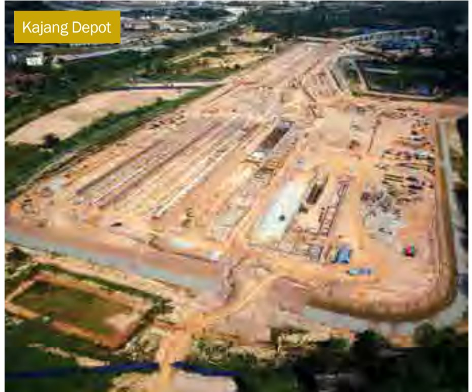
Building foundation, concreting and structural formwork in progress for the 60-acre Kajang Depot.
