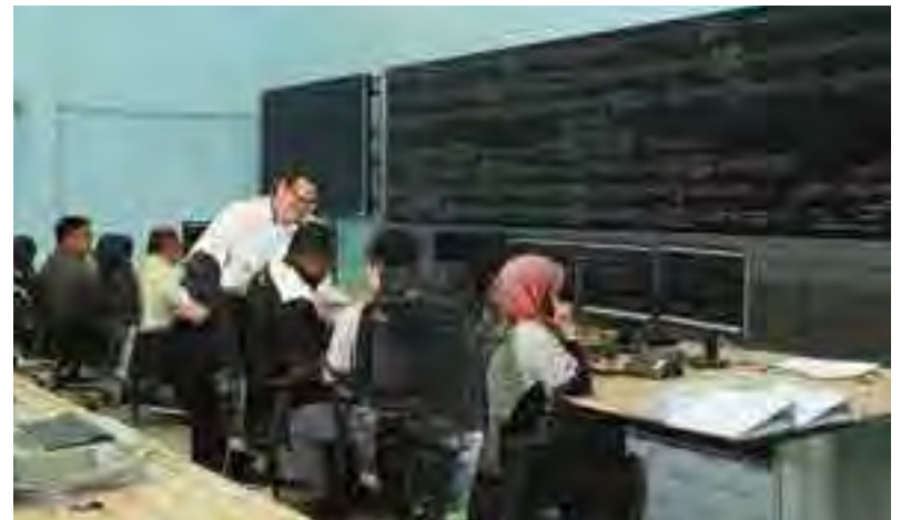
Picture shows the completed northern Centralised Traffic Control (CTC) located in Bukit Mertajam, Penang. It controls the railway signalling that centralised the train operations according to the railway system designated along the northern Electrified Double Track Project (Ipoh – Padang Besar).
