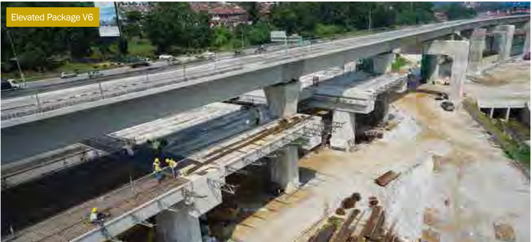
Six out of eight spans were completed for the concourse level of the future Taman Suntex MRT Station, along the Cheras-Kajang (Grand Saga) Highway.
