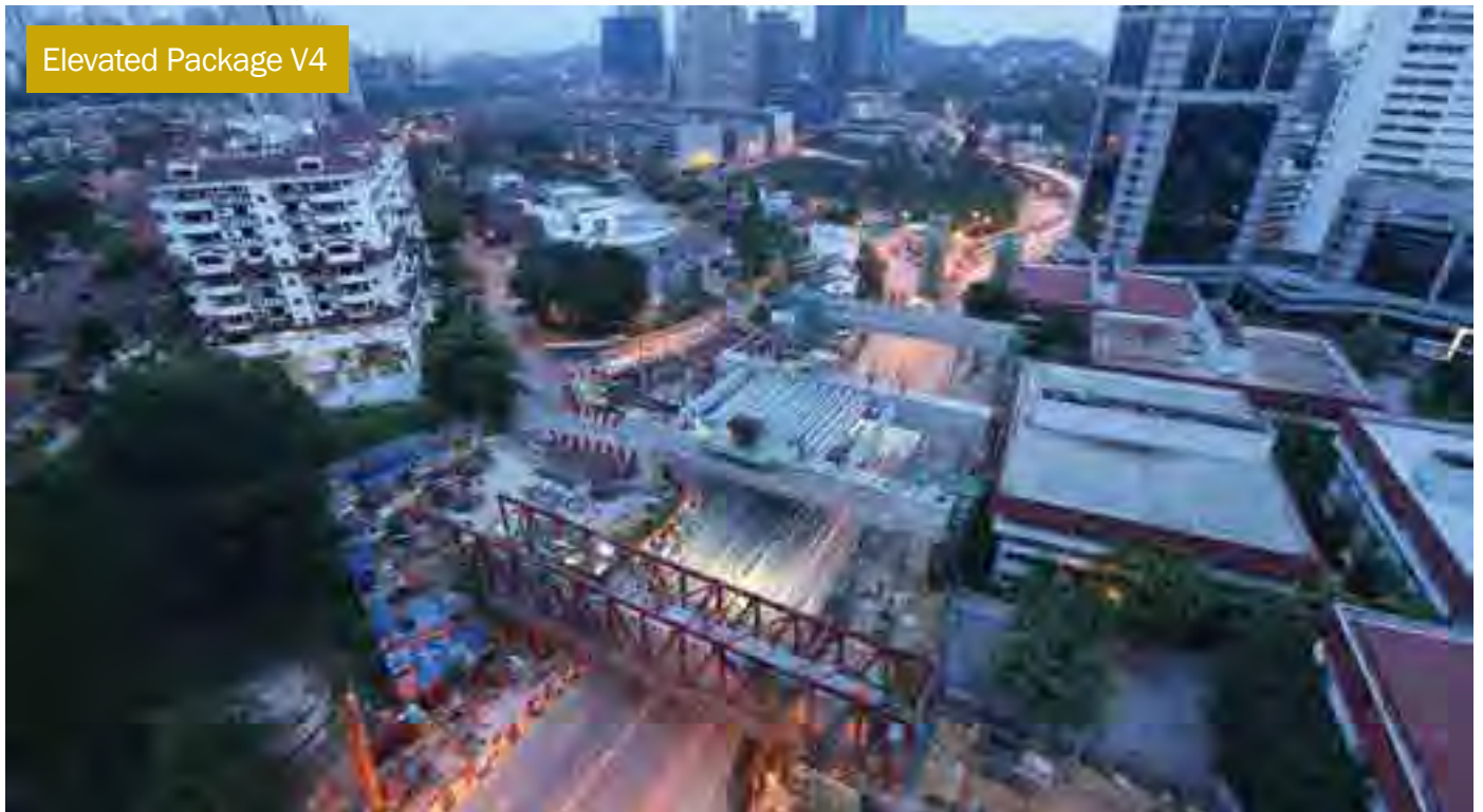
Beam launching and portal rebar works in progress for the future Semantan MRT Station, located along Jalan Semantan. Comprehensive traffic management plan was implemented to accommodate construction works amidst heavy traffic.
