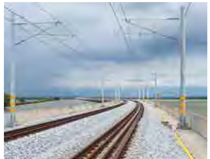
This completed 3.3km double track railway Bukit Merah Marine Viaduct, Perak, is replacing the existing single track railway causeway crossing Bukit Merah Lake.
