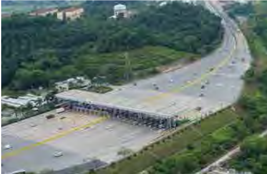
The Puchong Selatan toll plaza continues to see strong traffic growth as it is a crucial gateway to Putrajaya and Cyberjaya.
