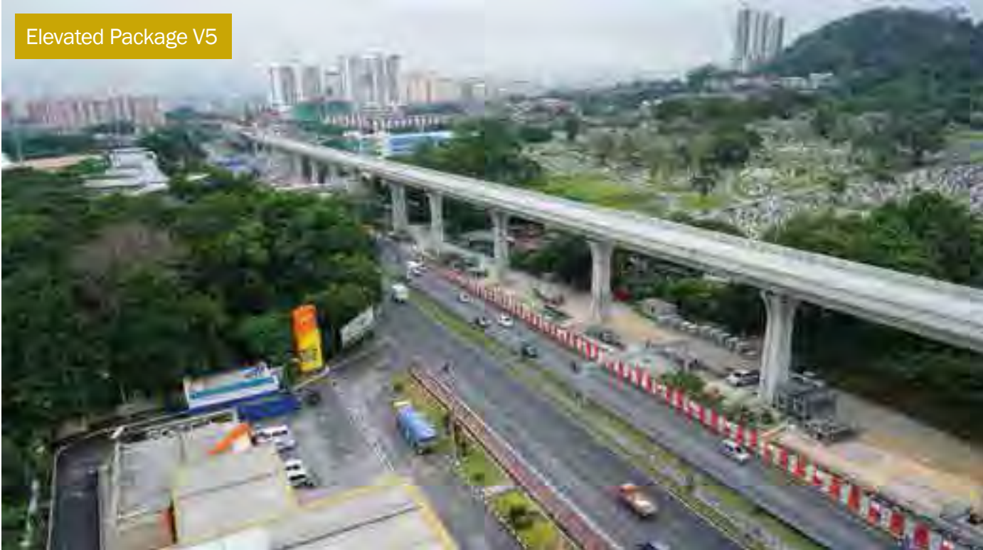
Completed MRT guideway with parapet wall installed along Jalan Cheras.
