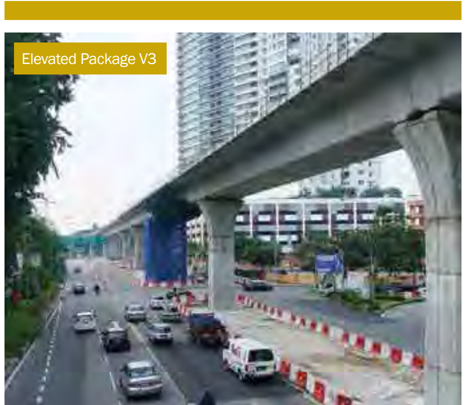
Parapet installation in progress for the completed MRT guideway along Jalan Damansara, passing Sinaran TTDI condominium at TTDI as the alignment heads towards TTDI MRT Station.
