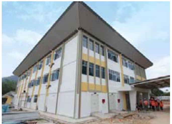
Signaling and Control systems are currently being installed at the Bukit Mertajam Centralised Traffic Control (CTC) facility, which will oversee and manage all railway operations within the Ipoh - Padang Besar double track project area, whilst communicating and synchronising train movements with the existing CTC at KL Sentral
