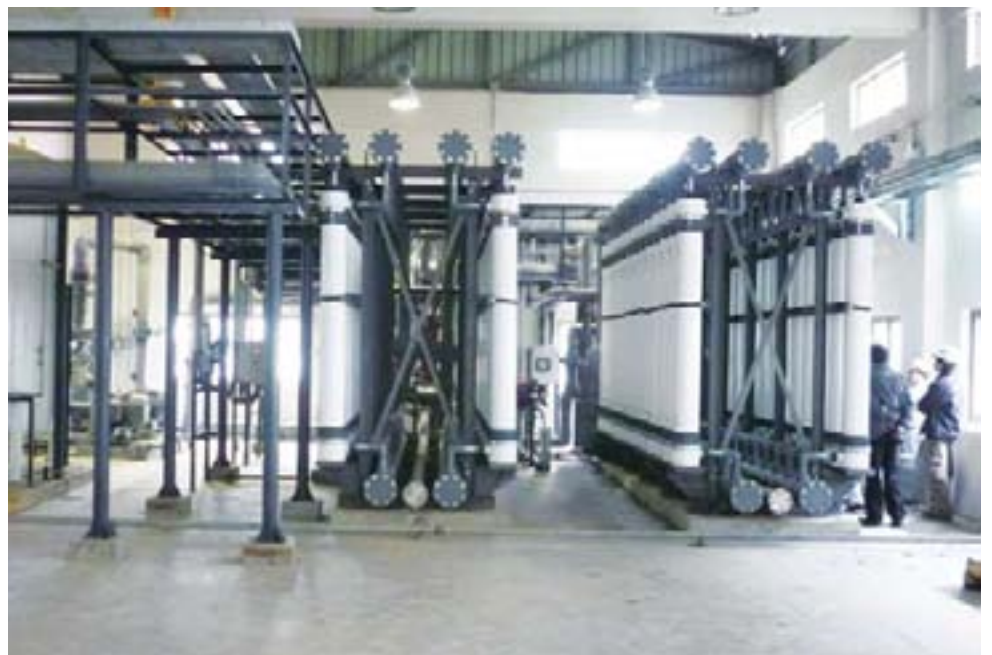
Part of the UV-treated water is channelled to undergo Membrane Filtration to further improve its clarity to render it suitable for recycling within the STP for non-potable use
