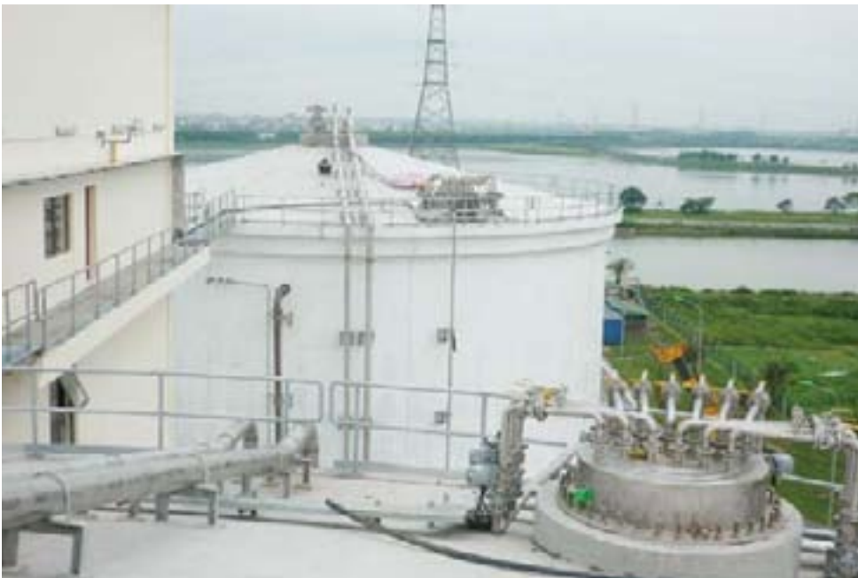
Sludge settled out from the Sequence Batch Reactor (SBR) tanks are sent for thickening and then to the anaerobic digester tanks (picture above) to be digested at a temperature of about 36°C for 20 days.
