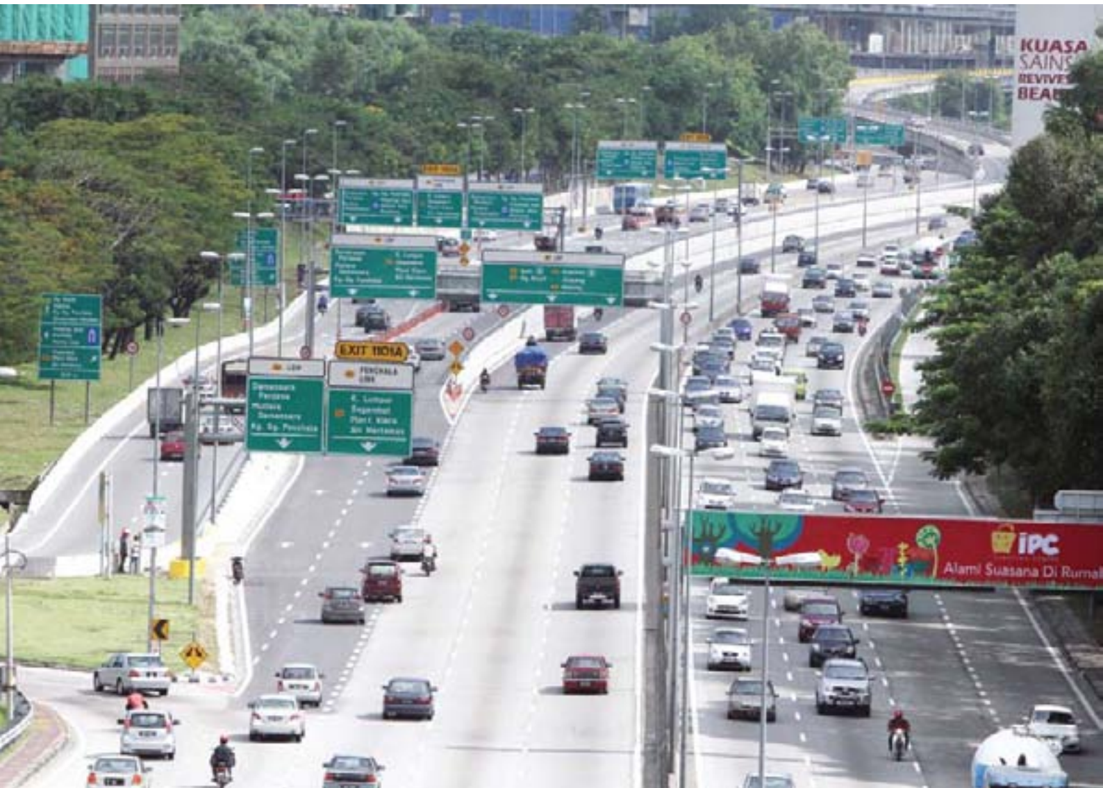
One of the three packages for the LDP 5 major upgrading initiative – Package B – involves upgrading works for Kepong-bound traffic on the Damansara - Puchong Highway (LDP) between Persiaran Surian and the Penchala Toll Plaza
