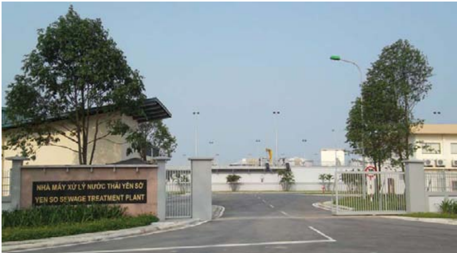
The Yen So Sewage Treatment Plant in Hanoi, which is currently in the final stages of handover, sits on a 23-acre piece of land, 7km south of the city
