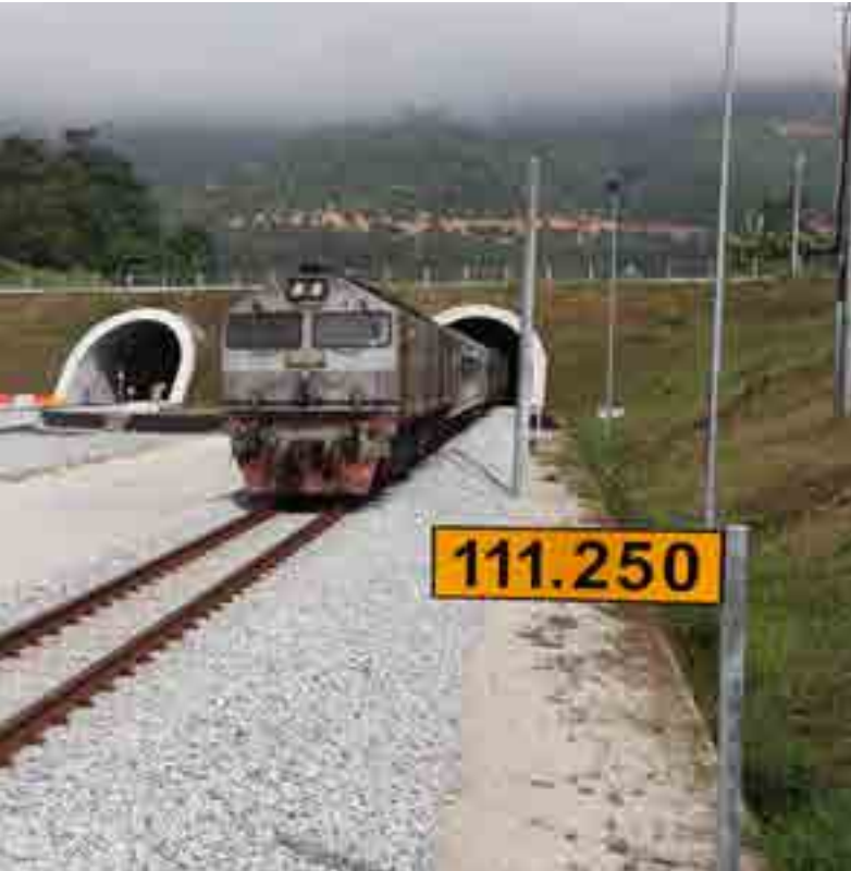
Picture shows a KTMB passenger train travelling from Butterworth to Kuala Lumpur passing through the newly commissioned 3.3km twin-bore Berapit Tunnel in the state of Perak.
