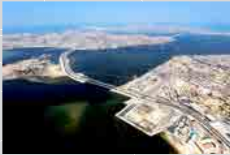
Sitra Causeway Bridges
