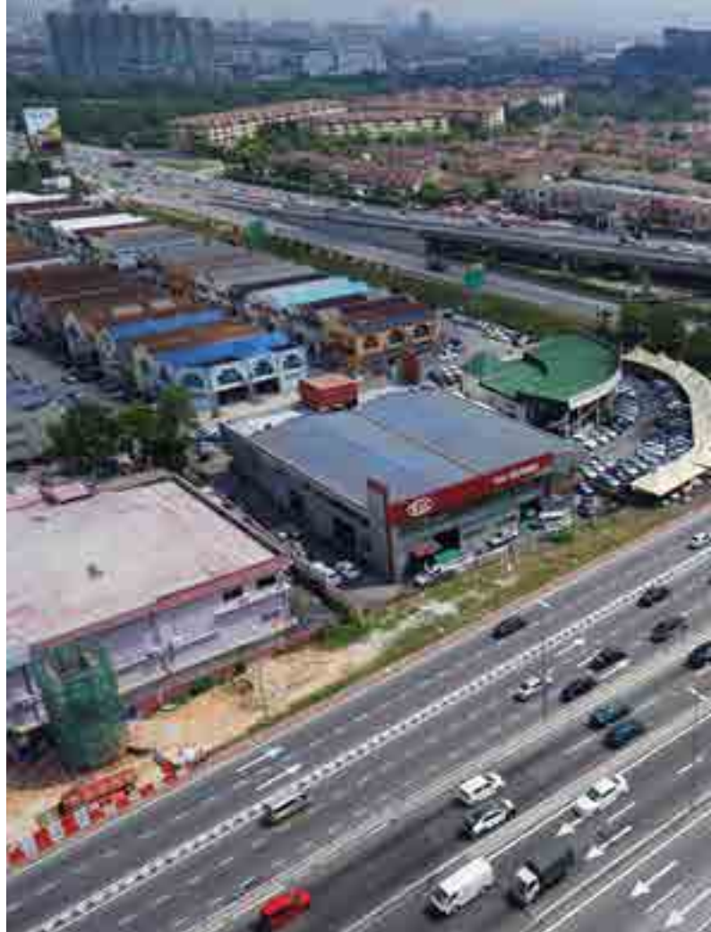
Aerial view of the widened LDP after the LDP 5 Package C upgrading works that runs from the Puchong Jaya Interchange towards Putrajaya and Shah Alam.
