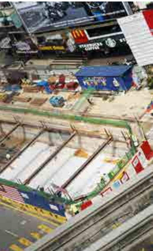
Aerial view of the Semantan Portal. Two Earth Pressure Balance Tunnel Boring Machines (EPB TBMs) were launched from this portal and tunnel towards the KL Sentral MRT station.
