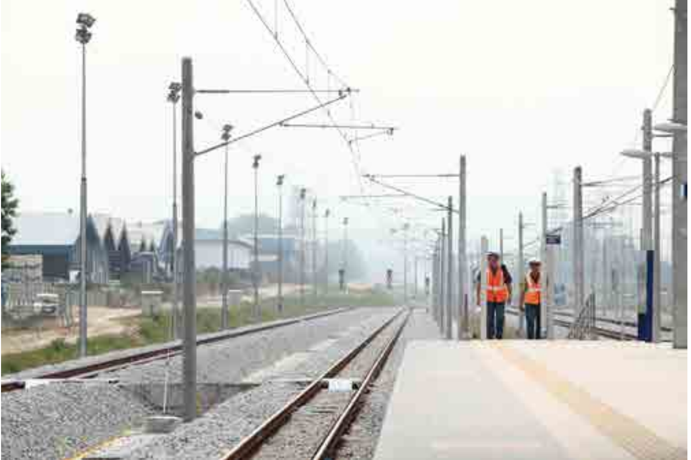
Picture shows completed track works at the new Tasek KTMB Station.
