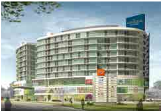
Artist impression of the Gamuda Biz Suites multi-storey commercial development in Kota Kemuning.
