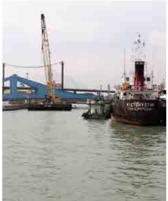
The newly-commissioned Prai Swing Bridge in Prai, Penang, serves as both a double railway track and a swing bridge that allows passage for passing marine vessels via its rotating mid-span.
