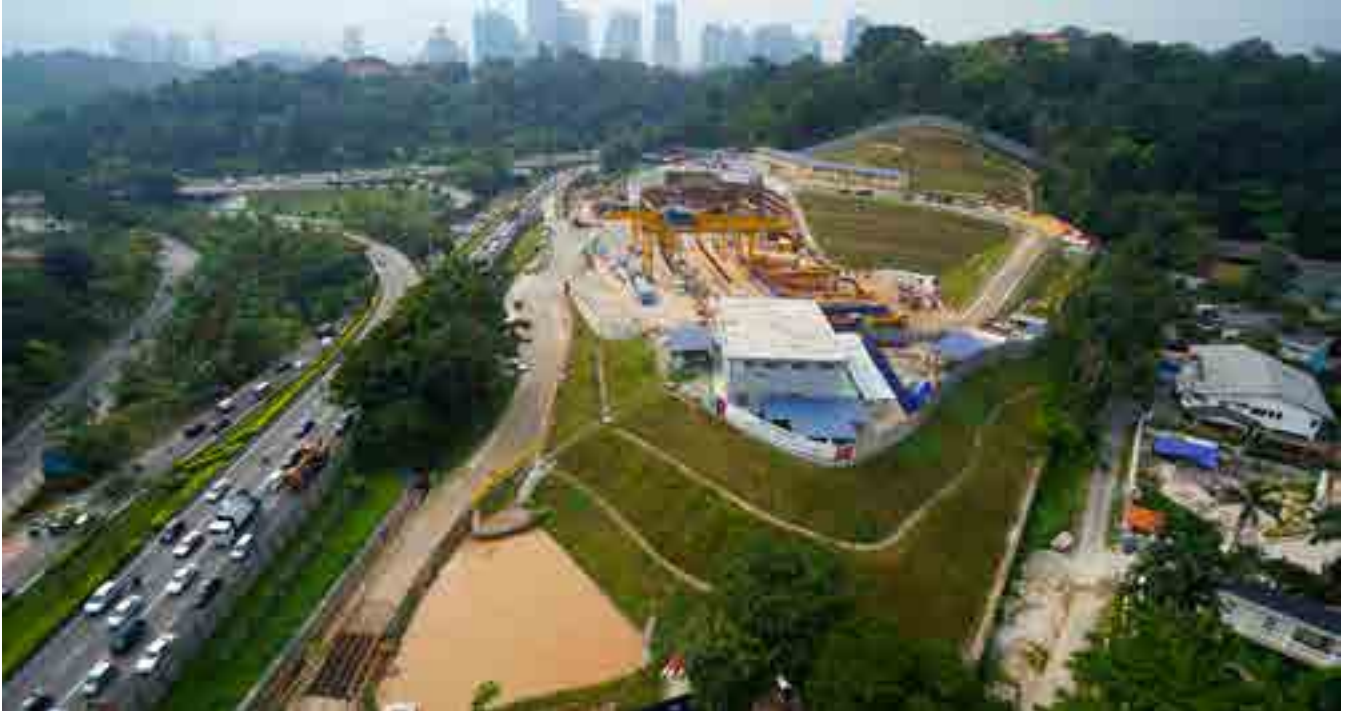
Aerial view of the Semantan Portal. Two Earth Pressure Balance Tunnel Boring Machines (EPB TBMs) were launched from this portal and tunnel towards the KL Sentral MRT station.
