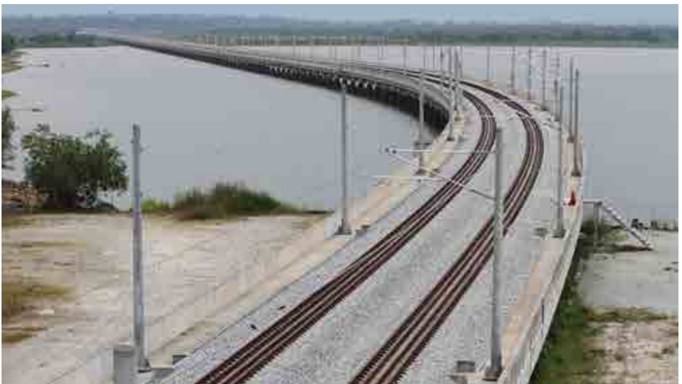
The 3.45km Marine Viaduct, built across the northern tip of the Bukit Merah Lake, will serve as the only above-water double railway track constructed for electrified high-speed trains in Malaysia.
