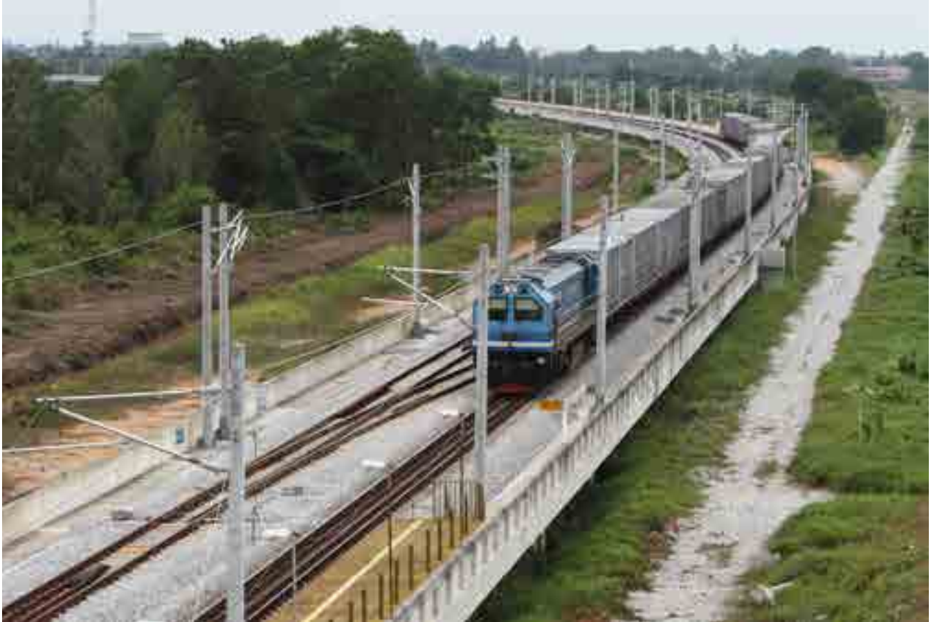
The 29km elevated Land Viaduct is specially designed to stay well above potential flood levels when the alignment runs past low-lying areas between Alor Pongsu and Parit Buntar in the state of Perak.
