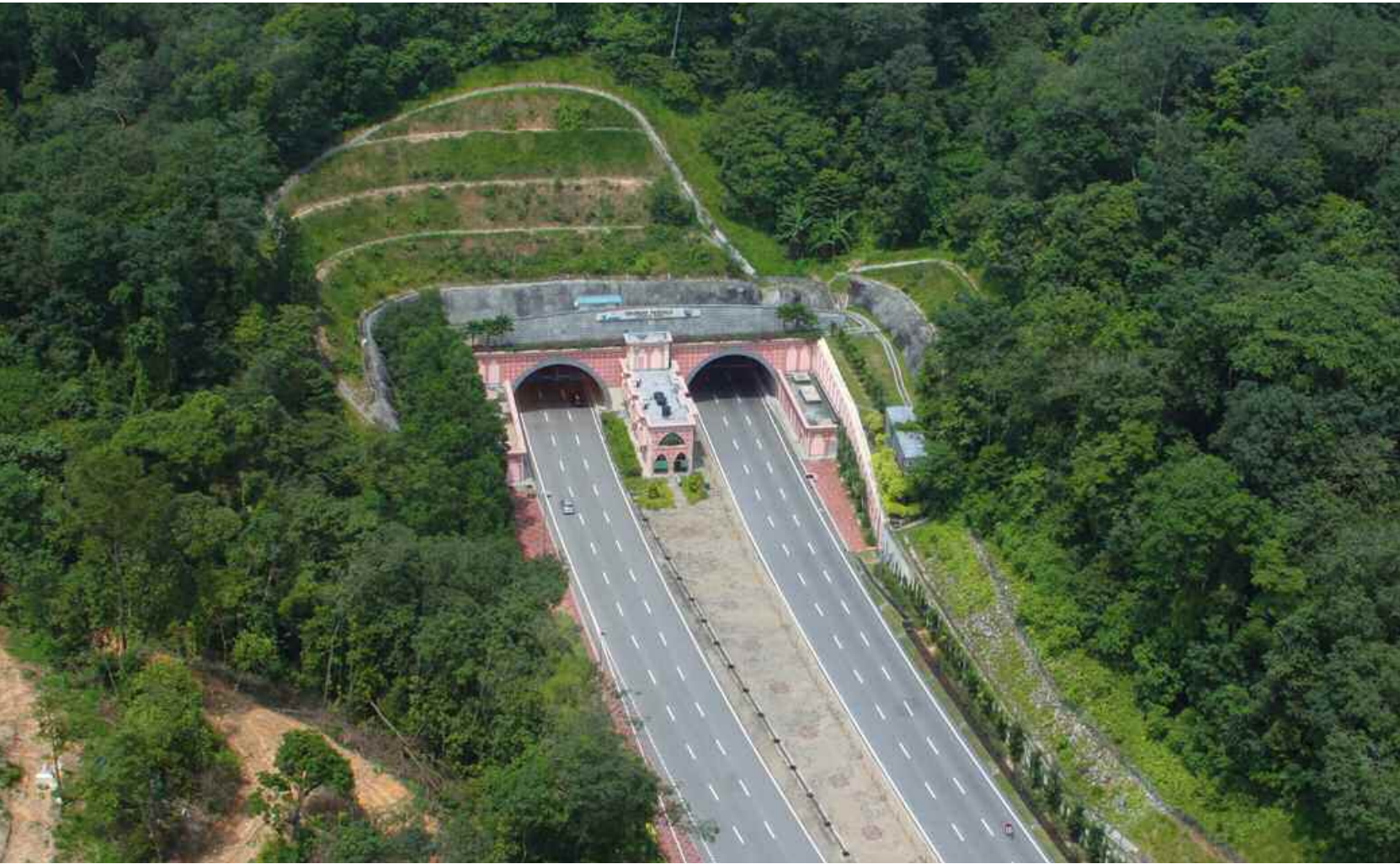
▲ Penchala Tunnel - a unique 710m twin bored tunnel
