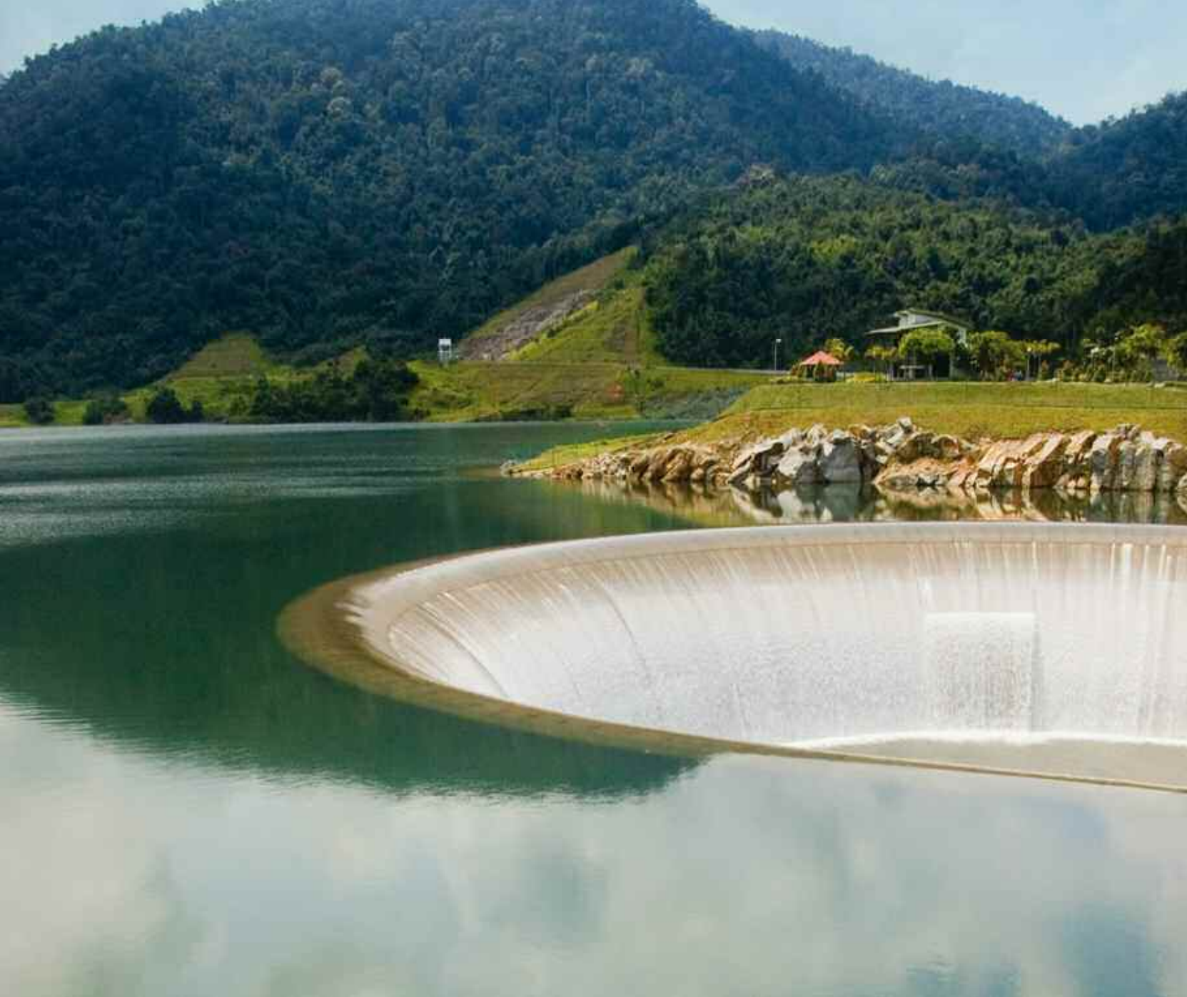
▲ Overflowing Sungai Selangor Regulating Dam
