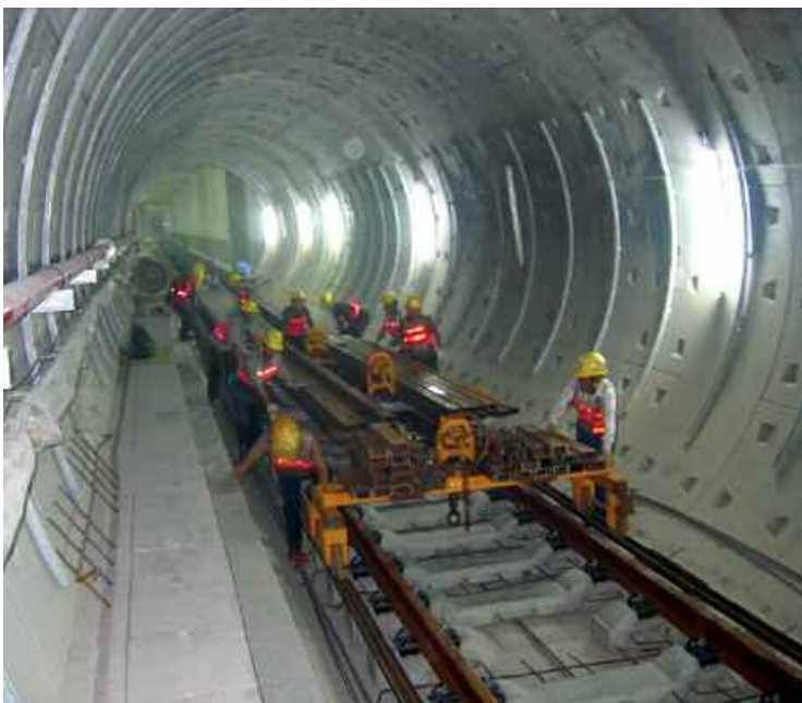
▲ Kaohsiung MRT - track laying works in progress
