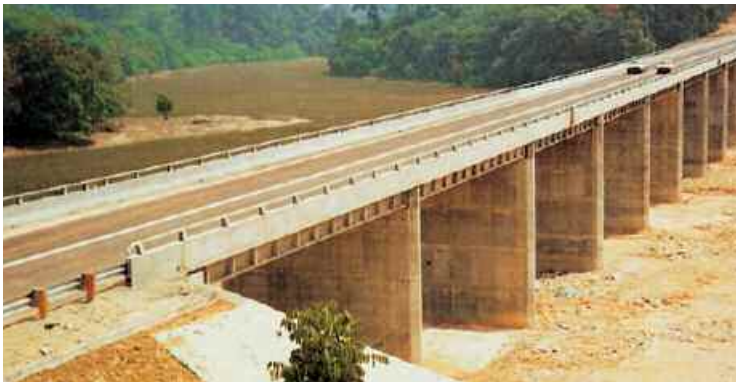
▲ Temerloh-Mentakab By-Pass, Pahang
