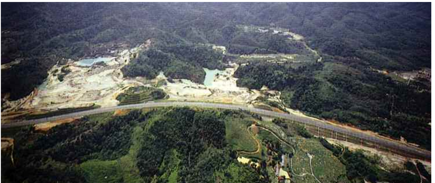
▲ Simpang Pulai - Gopeng Highway, North South Expressway
