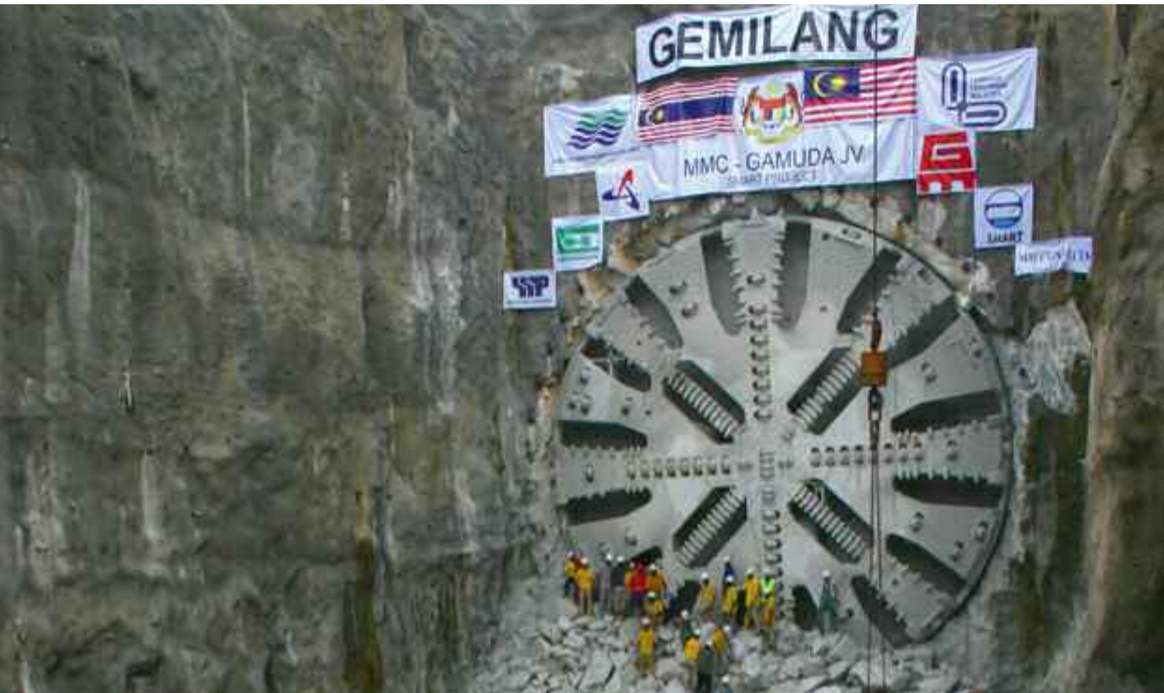
▲ SMART's TBM Gemilang tunnel breakthrough
