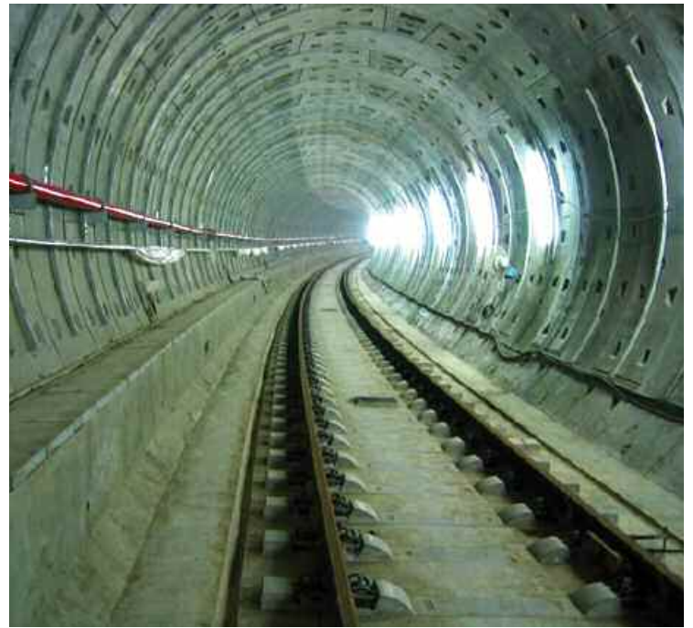
▲ Completed tunnel section of Kaohsiung MRT, Taiwan
