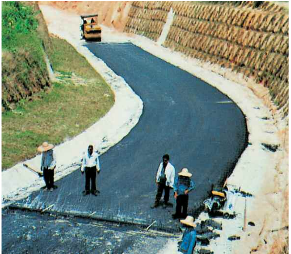
▲ Paving of access roads to Pergau Dam, Kelantan
