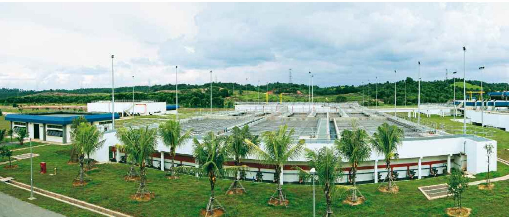
▲ Bukit Badong Water Treatment Plant
