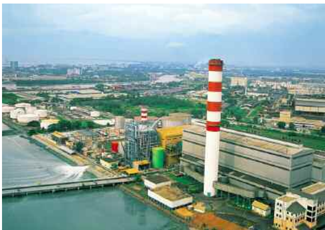
▲ Prai Power Station Phase II
