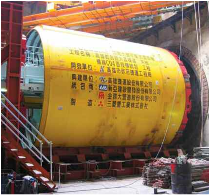
▲ Kaohsiung MRT's TBM involved tunnelling and deep excavation in soft soil
