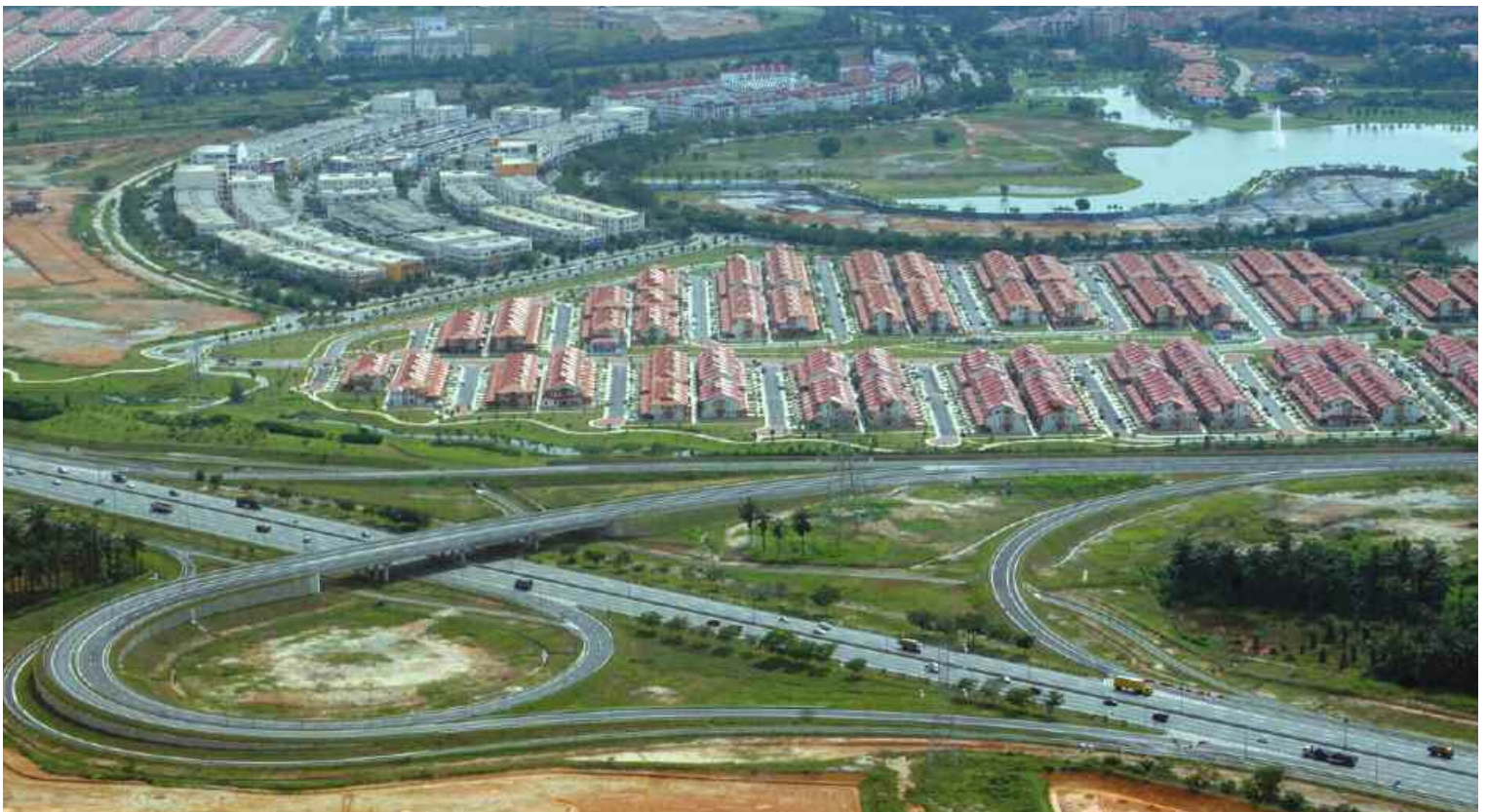
▲ Aerial view of Kemuning Interchange, Shah Alam Expressway - innovative surcharging methods were used in ground improvement works.
