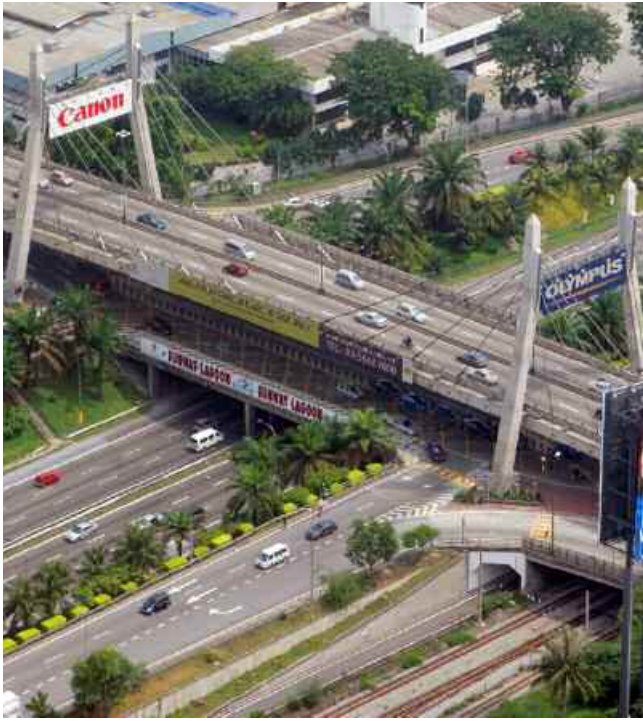
▲ Malaysia's first cable-stayed bridge over land at the LDP
