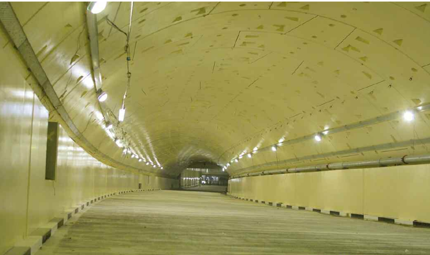
▼ SMART's motorway tunnel upper deck
