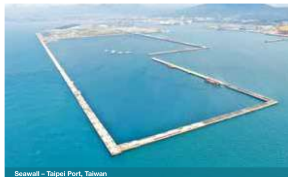
Seawall - Taipei Port, Taiwan
