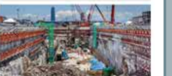
Construction site showing workers and equipment.
