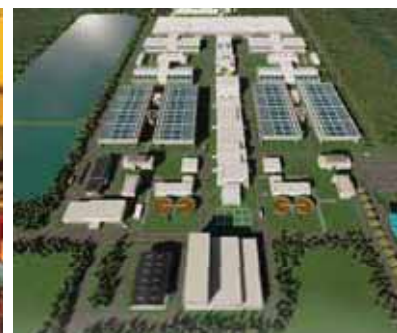
Rasau Water Treatment Plant - Selangor, Malaysia
