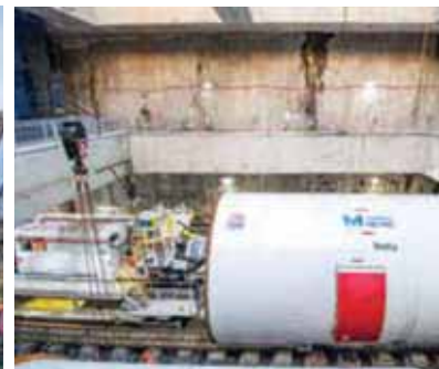
Sydney Metro West Tunnelling - Australia
