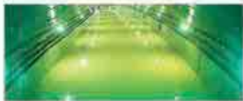
Inside SMART Tunnel during Mode 4.
