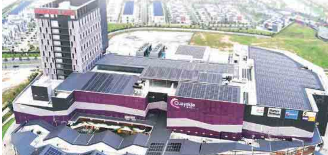
Solar PV installed at Quayside Mall, twentyfive.7.
