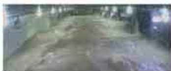
CCTV Images of the SMART Tunnel after activation.
